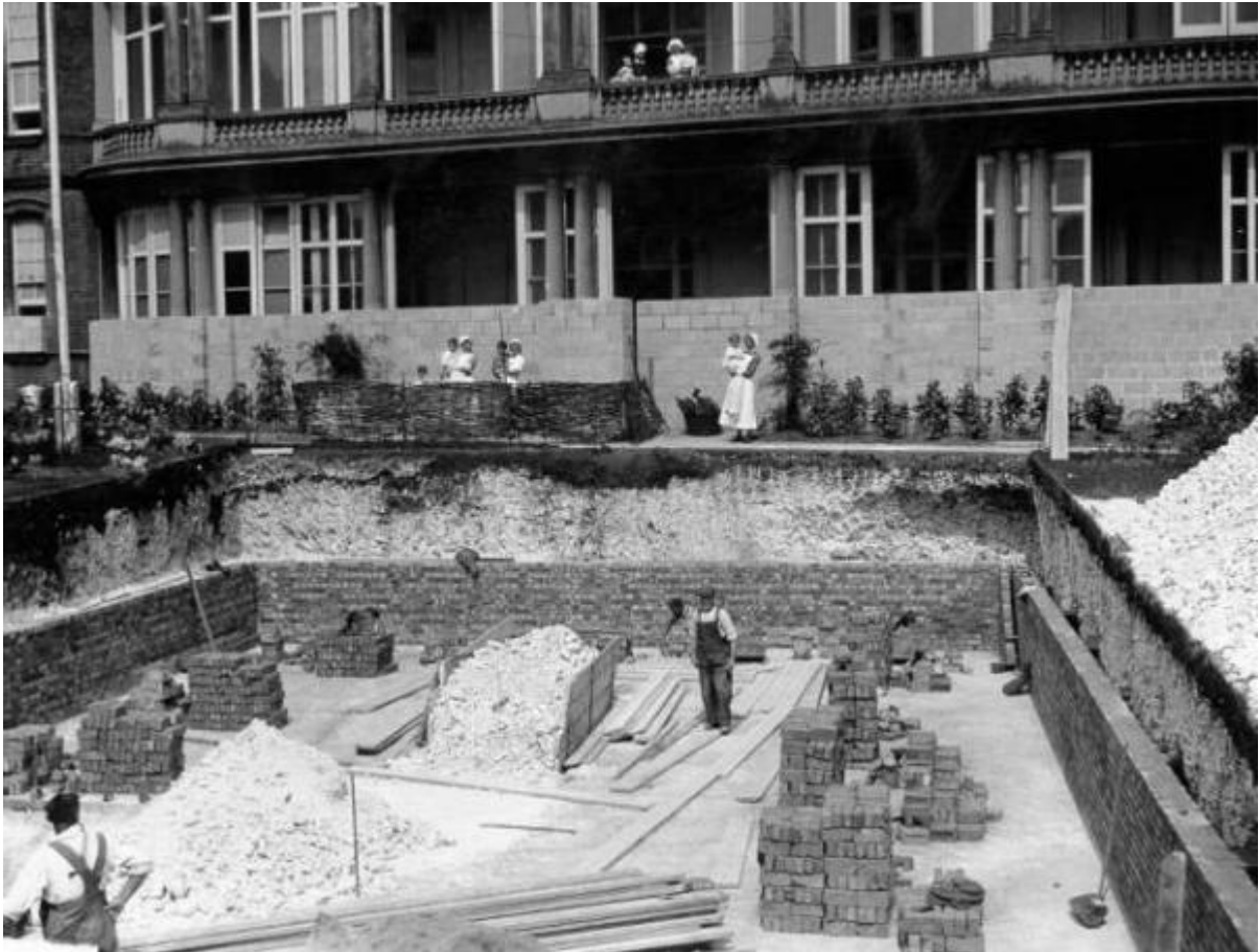
The building of an air raid shelter at the Royal Alexandra Hospital, c. 1938
