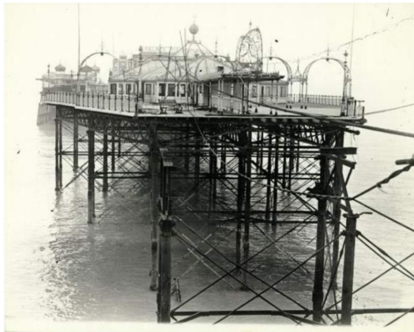
Gap in Palace Pier made in 1940 in case of German invasion. The pier was not repaired until September 1945, four months after V.E. Day. All Sussex piers were cut in half and heavily mined for the duration of the war.
