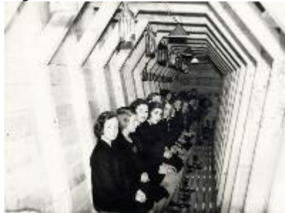
Roedean Tunnel Air Raid Shelter for Roedean School, c. 1939 Brighton and Hove in Pictures
