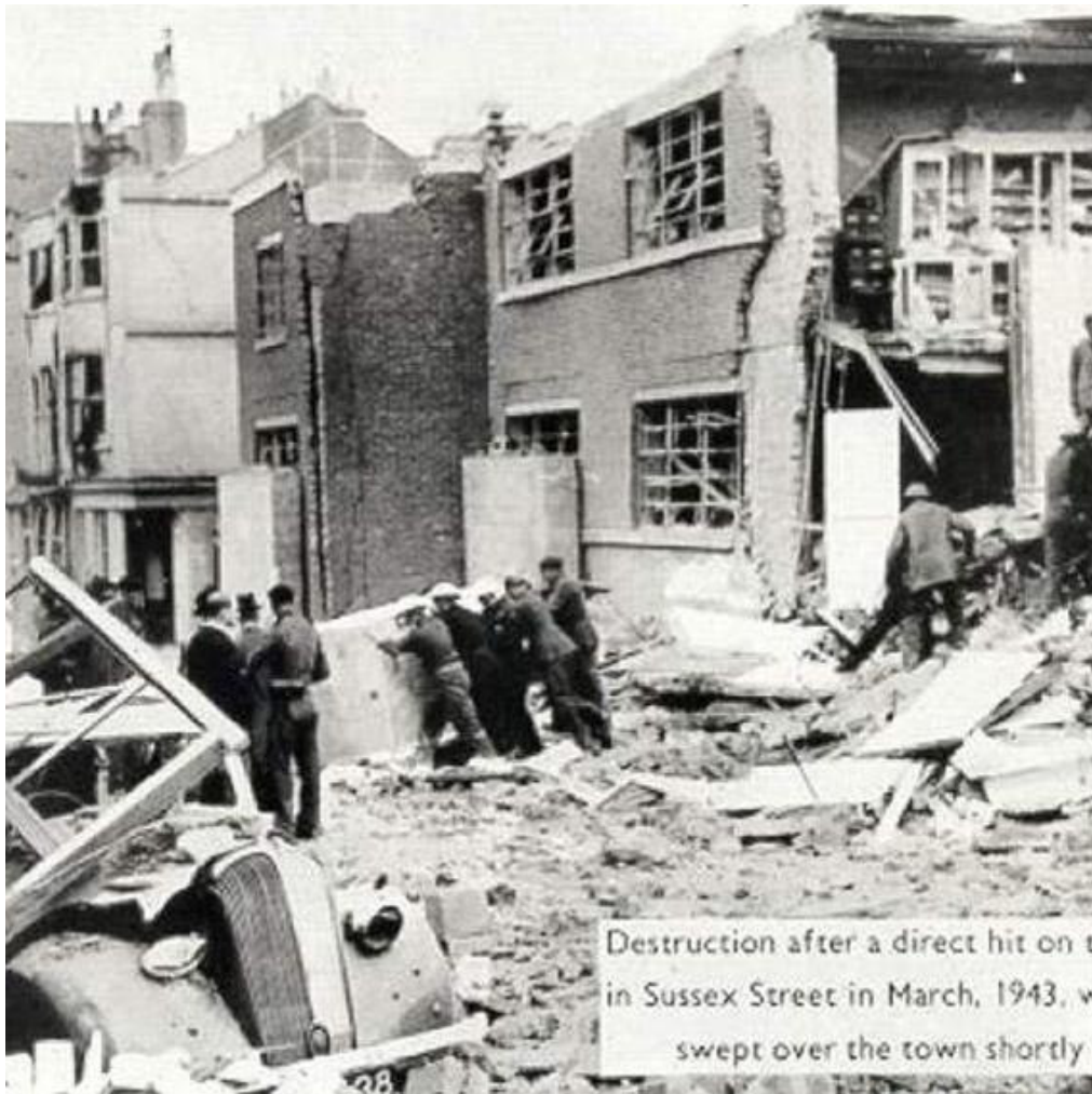
Bomb damage in Sussex Street, 1943
