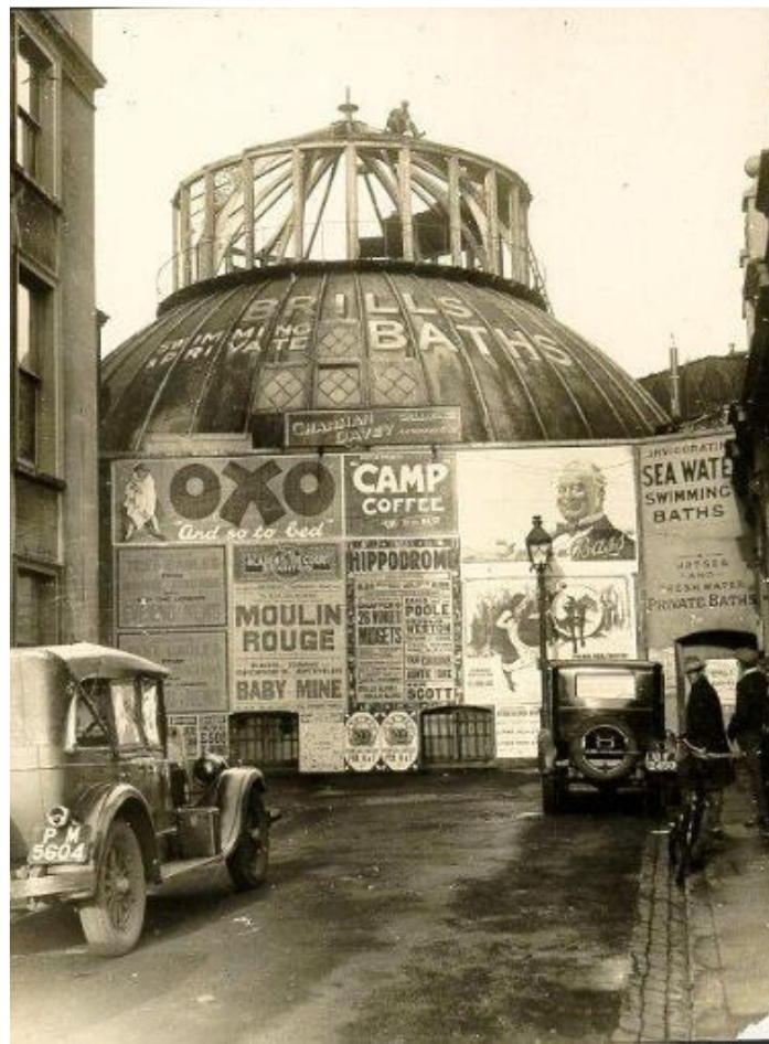
Brill's Baths in the course of its demolition in 1933. With wall of advertisements for OXO, Camp Coffee, Bass and performers at the Academy and The Court and The Hippodrome.
